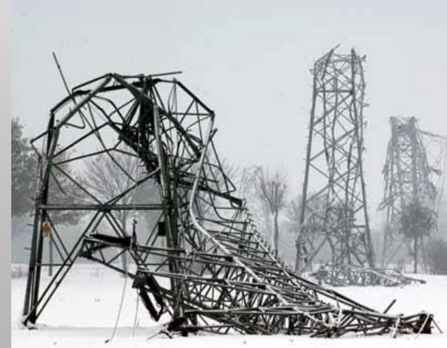
Failure of power line masts caused by extreme ice packages (BAM)
