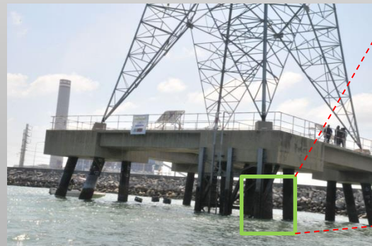
Larger aggression of marine waters due to climate changes entail significant corrosion in the splash water zone of high-power transmission systems (MTec)
