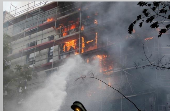
Fire at polystyrene insulated front of a residential building ( www.feuerwehr.de )
